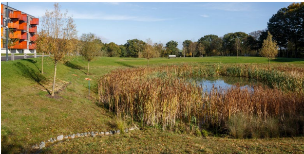
Image 23: Example of attenuation pond / Source: Essex SuDS design guide
